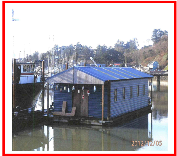
The new float house
